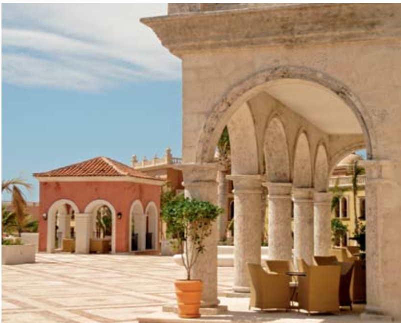
From top: A preview of what's to come at Sotogrande at Cap Cana. Inside one of the spacious luxury villas in Caletón at Cap Cana. The just-opened Sanctuary Cap Cana Golf & Spa boasts interesting architecture, a multitude of dining and entertainment options, luxe accommodations, and a prime oceanfront location.
